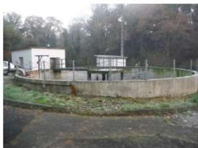
Photo 11 : Silo de stockage à boues de 300 m<sup>3</sup>
